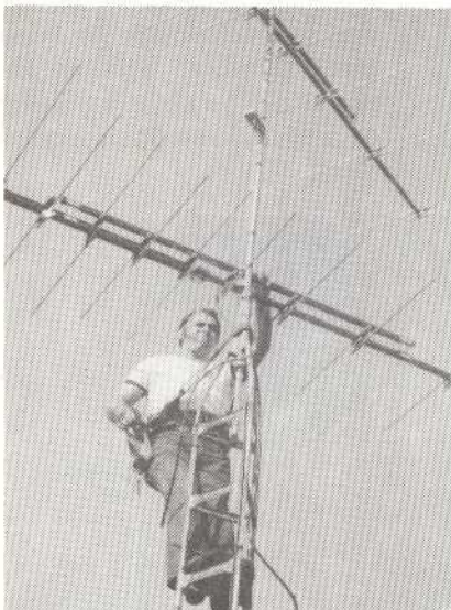
The lower antenna is mounted approximately 72" below upper antenna.
