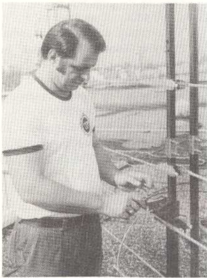
After connecting a 52' length of CL-2700 to the output of the terminal board, Rabong screws the housing shut.
