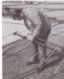
The CH-6060 features a double-boom for additional strength. Rabong attaches the two together with a heavy-duty brace.
