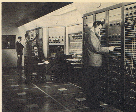
The Master Control Board in the Radio Canada Building in Montreal is the nerve center of the CBC's broadcasting installation. It can handle five transmitter feeds, eight outgoing networks, seven incoming networks, 23 studios, and was designed for one-man operation. The switching of all circuits is performed by remotely-controlled relays.
