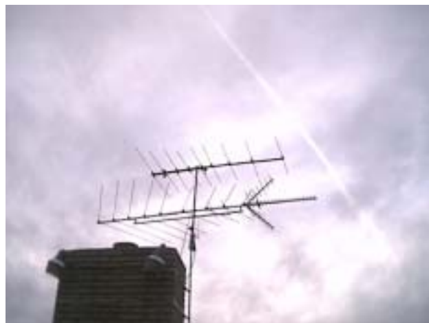
Kevin Redding's Antenna System in Mesa, Arizona
