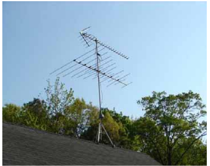
Jeff's antennas: Winegard PR-9032 corner reflector top, PR-5030 bottom
