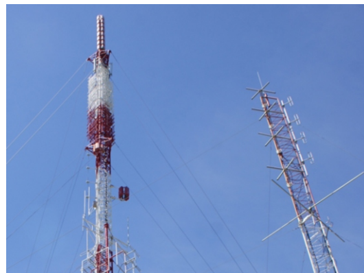
Broadcast towers located in Ciudad Habana. The tower on the left has been identified as primarily a TV broadcast tower, while the tower on the right has a variety of radio equipment.
