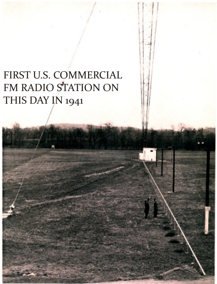
W47NV, Nashville: The FM antenna is atop the vertical radiator of WSM. This view shows the newly installed coaxial cable which feeds the FM turnstile. With the official inauguration of the FM transmitter, this station has undertaken a campaign to develop its FM audience, and to interest those within its coverage area in the purchase of A-FM receivers. WSM, a clear channel station, is one of the most influential and highly-regarded stations in the South.
