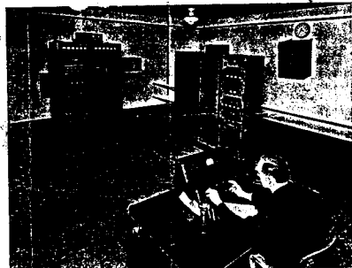
MASTER CONTROL ROOM OF THE FM STATION OPERATED BY THE BOARD OF EDUCATION
